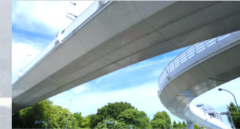
Large-scale Refurbishments of Three NEXCO Companies
