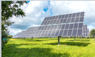
Solar Power Generation
