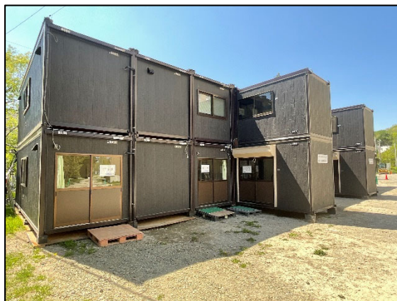
Exterior of construction office
