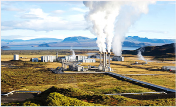
Geothermal Power Generation
