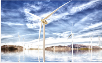
Wind Power Generation
