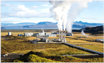
Geothermal Power Generation
