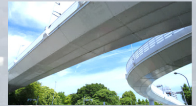
Large-scale Refurbishments of Three NEXCO Companies
