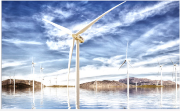
Wind Power Generation
