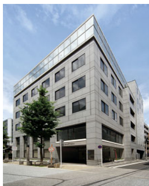
Tokyo Division Headquarters
