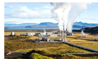
Geothermal Power Generation
