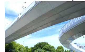
Large-scale Refurbishments of Three NEXCO Companies
