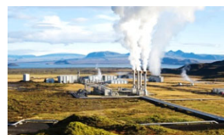
Geothermal Power Generation
