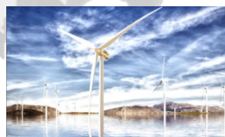
Wind Power Generation
