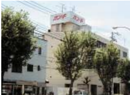
Kanki Corporation head office
