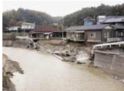
Site of riverbank collapse caused by Typhoon No. 23 (Kagawa Prefecture)
