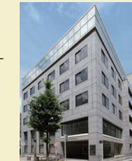
Kanamoto Hamamatsucho K Building (Business Coordination Headquarters)
