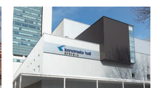
Kanamoto Hall (Sapporo Civic Hall) Housing a Large 1,500-person Event Hall as well as Small, Medium and Large Conference Rooms
