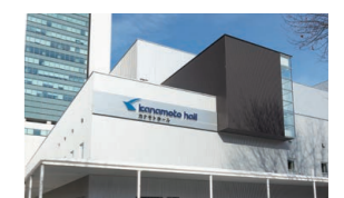
Kanamoto Hall (Sapporo Civic Hall) Housing a Large 1,500-person Event Hall as well as Small, Medium and Large Conference Rooms
