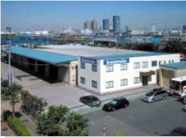
Shin-Kiba Branch / Shutoken Aerial Equipment Branch
