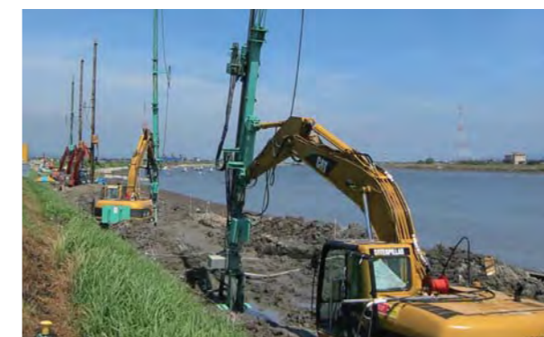
フローテクノ社の地盤改良機械 Flowtechno Corporation ground improvement equipment
