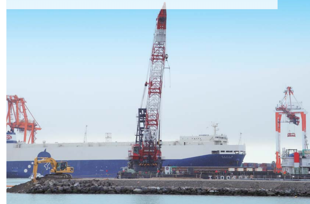
仙台塩釜港（宮城県仙台市）の岸壁築造工事 Bulkhead wharf construction works at Sendai-Shiogama Port (Sendai, Miyagi Prefecture)
