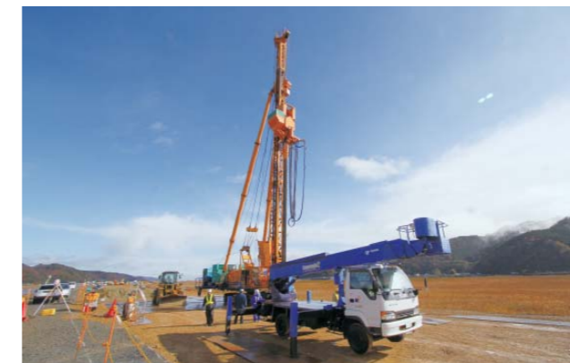
北上川（宮城県石巻市）の護岸工事 Bank protection works at Kitakamigawa (Ishinomaki, Miyagi Prefecture)
