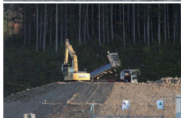
上：宮城県石巻市の護岸工事 下：宮城県南三陸町の高台造成工事 Top: Revetment works at Ishinomaki City, Miyagi Prefecture Bottom: Elevated land construction work in Minamisanriku, Miyagi Prefecture
