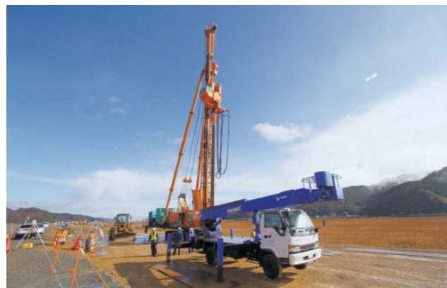
護岸や幹線道路などの地盤改良工事 Ground improvement works for projects such as seawalls and highways
