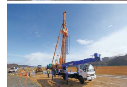
護岸や幹線道路などの地盤改良工事 Ground improvement works for projects such as seawalls and highways
