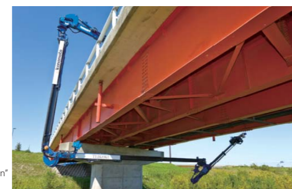
当社の橋梁点検車「橋竜」 Kanamoto's "Bridge Dragon" bridge inspection vehicle
