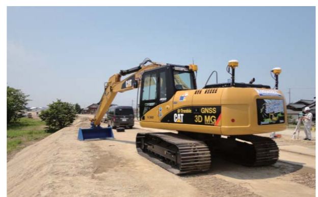
国土交通省が推進する情報化施工の現場 Site using information-aided construction technique promoted by the Ministry of Land, Infrastructure, Transport and Tourism
