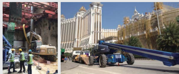
シンガポール（左）とマカオで進む大型プロジェクト Large-scale projects are under construction in Singapore (left) and Macau
