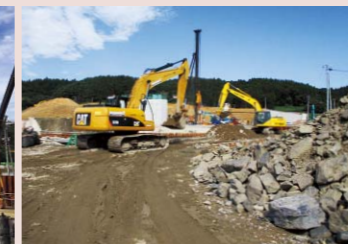
宮城県気仙沼市の復興道路整備工事 Reconstruction road construction work in Kesennuma City, Miyagi Prefecture
