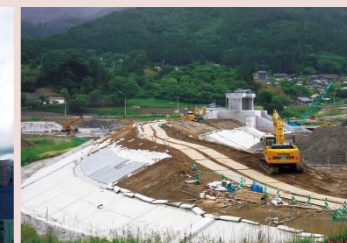
岩手県大船渡市の防潮堤工事 Coastal surge barrier construction works in Ofunato City, Iwate Prefecture
