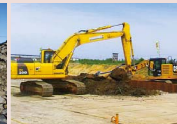
宮城県岩沼市の岩沼浜緑地工事 Iwanuma beach green land park construction works in Iwanuma City, Miyagi Prefecture
