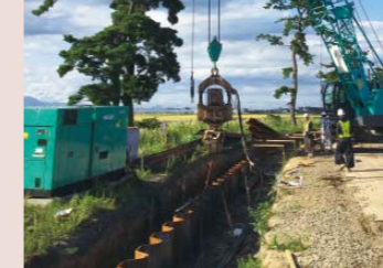
宮城県岩沼市の五間堀川河川災害復旧工事 Gokenbori River disaster restoration works in Iwanuma City, Miyagi Prefecture
