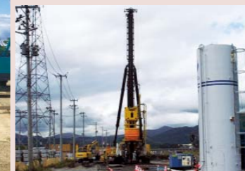
岩手県大船渡市の盛川道路改良工事 Morigawa Road Improvement works in Ofunato City, Iwate Prefecture
