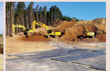
宮城県石巻市の防災集団移転工事 Disaster prevention collective relocation works in Ishinomaki City, Miyagi Prefecture
