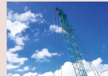
宮城県牡鹿郡女川町の国道398号新設工事 New construction works on National Highway 398 in Onagawa Town, Oshika-gun, Miyagi Prefecture
