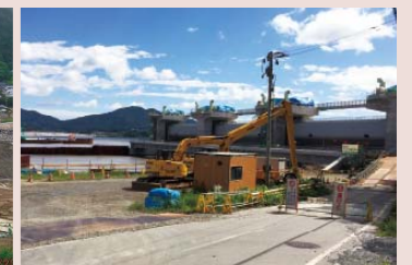
岩手県陸前高田市の気仙川の水門新設工事 Kesen River flood gate construction works in Rikuzentakata city, Iwate Prefecture
