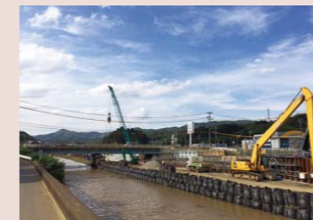
宮城県気仙沼市の河川外災害復旧工事 Riverbank restoration work in Kessanuma City, Miyagi Prefecture
