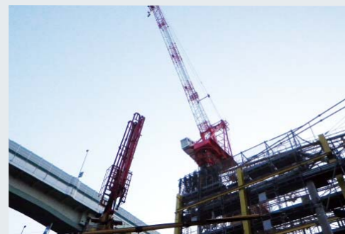
首都高速道路の耐震補強工事 Tokyo Metropolitan Expressway seismic reinforcement works
