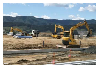
岩手県陸前高田市の高台造成工事 High ground construction work in Rikuzentakata City, Iwate Prefecture
