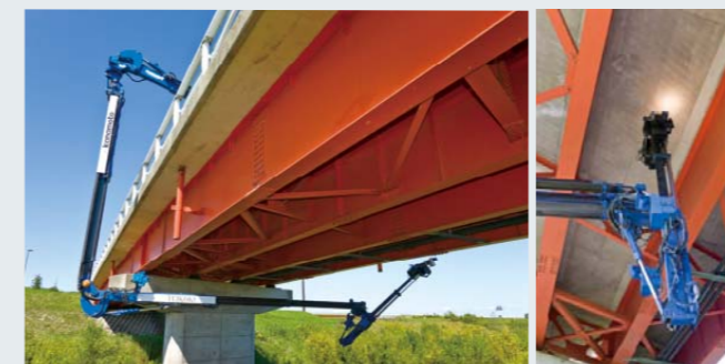
当社の橋梁点検車「橋竜」 Kanamoto's "Bridge Dragon" bridge inspection vehicle
