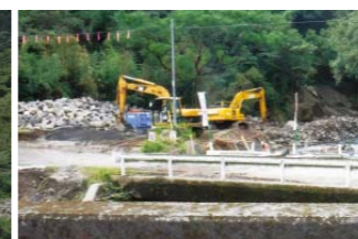
鹿児島県鹿屋市の河川災害復旧工事② River disaster restoration works in Kanoya City, Kagoshima Prefecture ②
