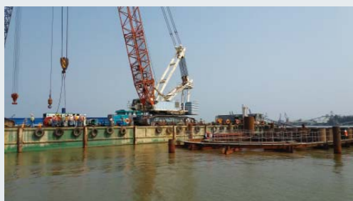
ベトナムで進む大型プロジェクト Large-scale projects are under construction in Vietnam
