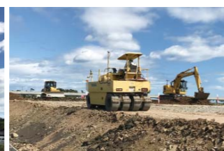
宮城県名取市の道路築造工事 Road construction works in Natori City, Miyagi Prefecture
