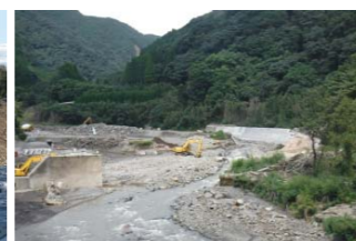
鹿児島県鹿屋市の河川災害復旧工事① River disaster restoration works in Kanoya City, Kagoshima Prefecture ①
