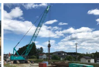
宮城県亘理郡山元町の護岸工事 Bank protection works in Yamamoto Town, Watari-gun, Miyagi Prefecture
