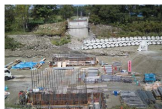
北海道河西郡芽室町の上芽室橋災害復旧工事 Memuro bridge disaster reconstruction works in Memuro Town, Kasai-gun, Hokkaido
