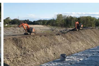
北海道河西郡芽室町の河川災害復旧工事 River disaster restoration works in Memuro Town, Kasai-gun, Hokkaido
