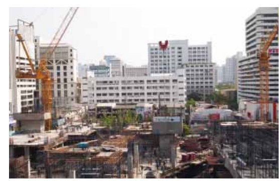
タイで進む再開発の建設工事現場 Construction site for redevelopment to advance in Thailand
